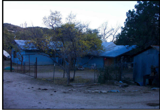
Photo [2] – Main ranch house
