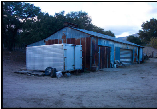
Photo [3] – Metal shop building
