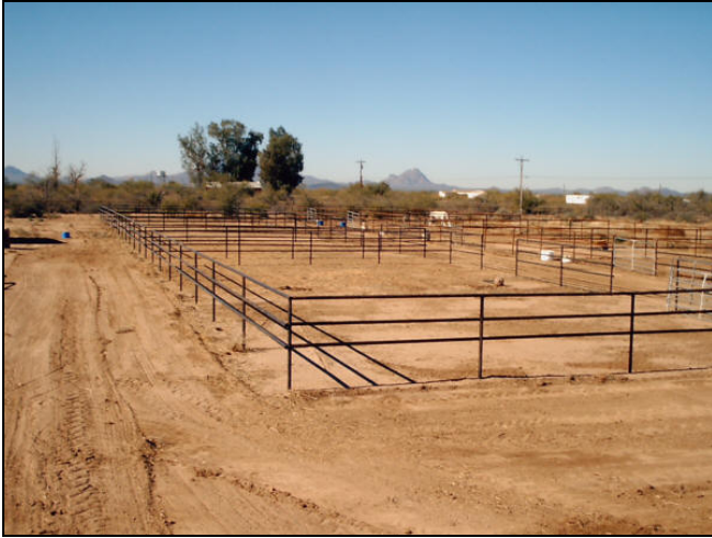
Photo [2] - Turnouts under construction
