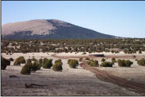
[2] Steel storage tank
