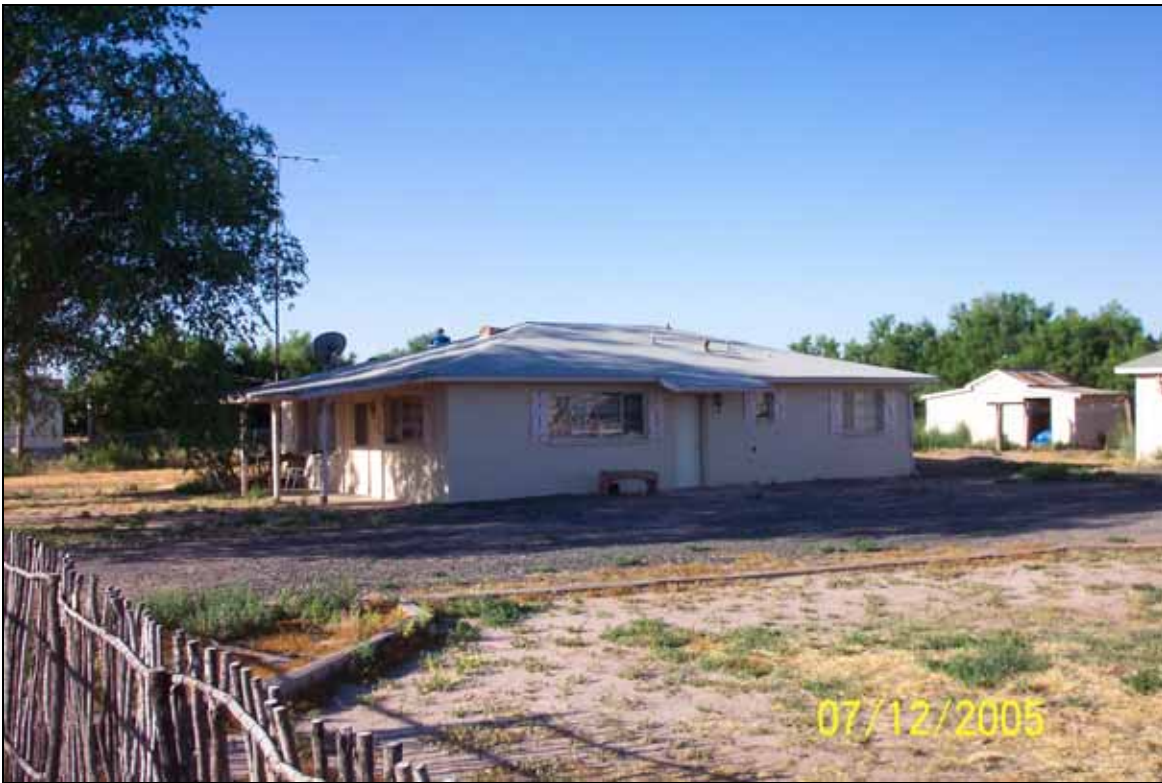
[3] Concrete Block Bunkhouse
