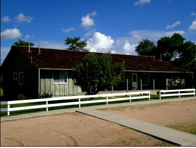
The guest duplex at the Headquarters with the Colt and Winchester suites.
