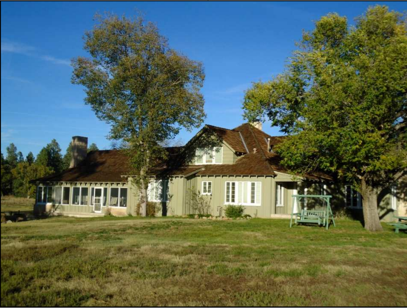
The owner's residence at the Headquarters.
