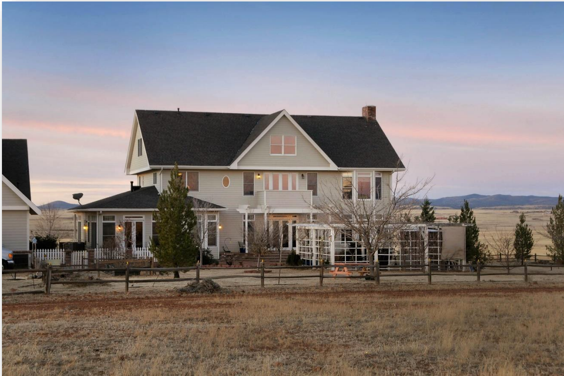
Rear View of Main House with Pergola
