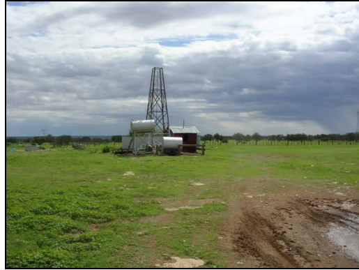
[3] Headquarters well & generator
