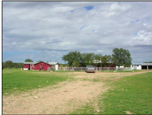
[5] Residence and storage sheds
