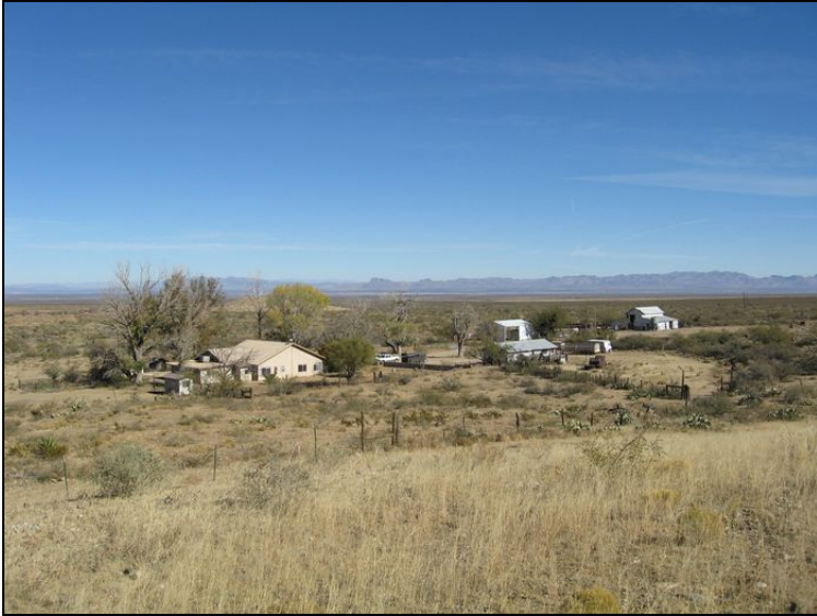
View of Headquarters Improvements
