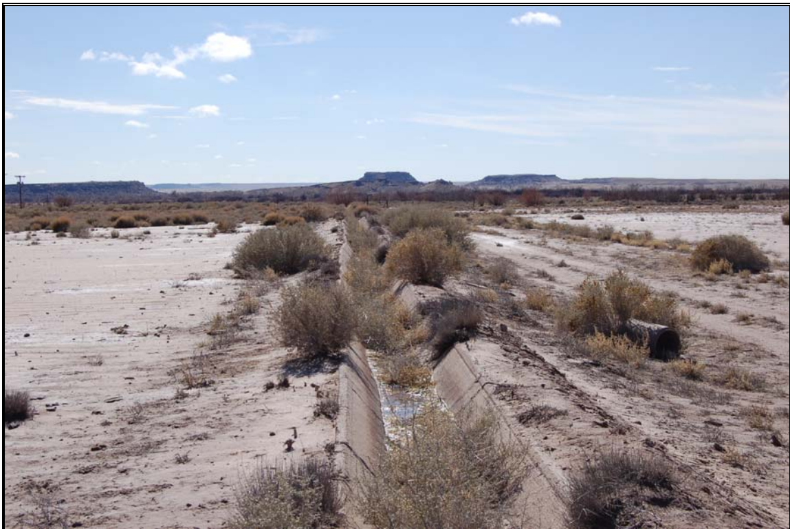
Concrete ditch for one of the fields.
